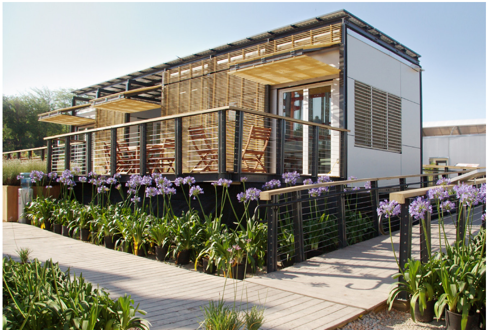
Completed project RE:FOCUS stands ready for viewing in the Solar Village in Madrid, Spain
